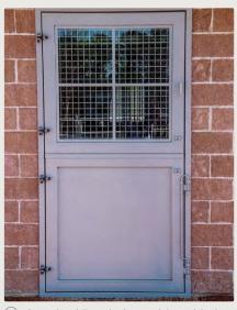
F Standard Dutch door with welded insert and mesh window guard
