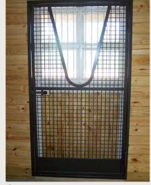
(H) Mesh stall screen and yoke opening and metal shaving guard
