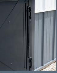
Cane-style door latch safely secures the door close
