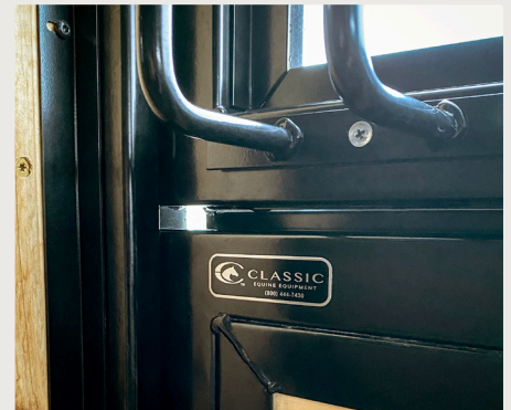
Dutch door has no protruding parts on the interior to snag
